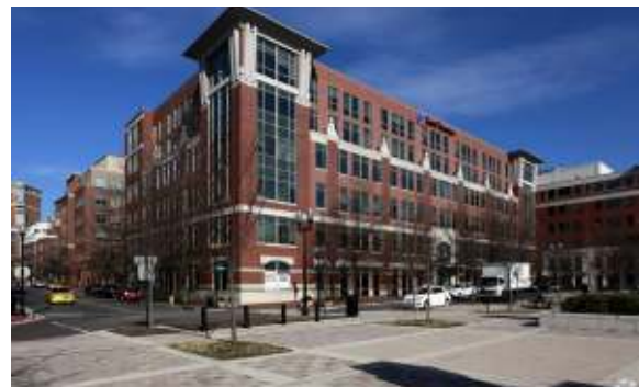
333 John Carlyle Street: new 64,614 SF office home for NCMEC after the organization vacates their prior headquarters at 699 Prince Street.
